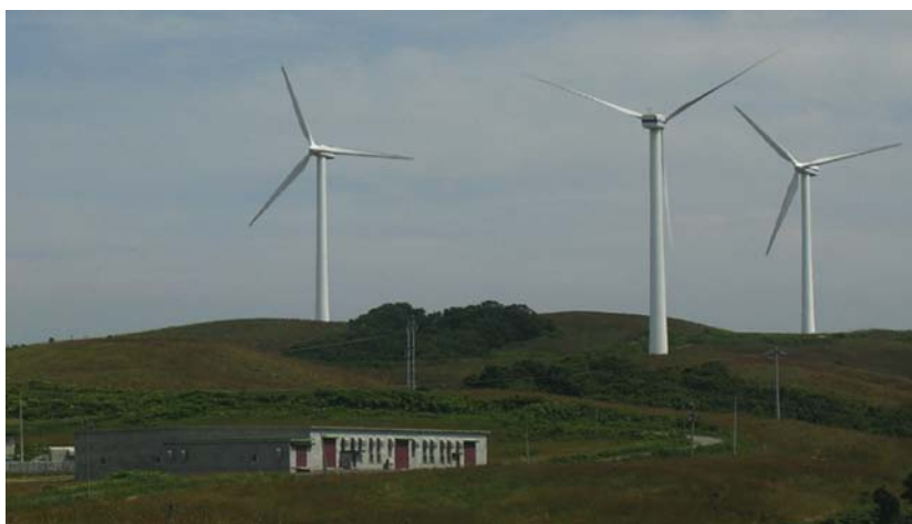
37. Experimental 4 MW, 6 MWh battery at Tomamae Villa wind park, Hokkaido, Japan.
